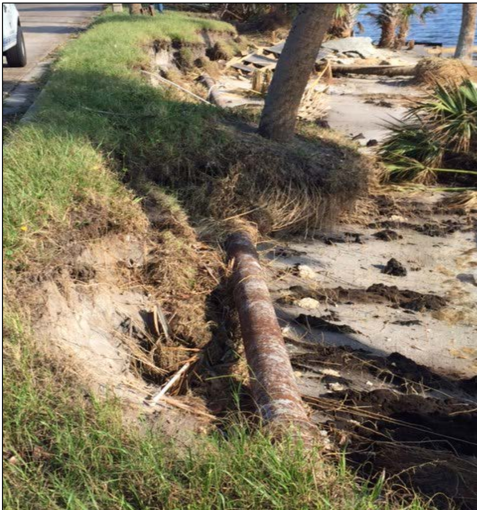
This image shows how erosion and flooding can begin to impair the integrity of roadways long before inundation occurs and also cause damage the underground utilities.
