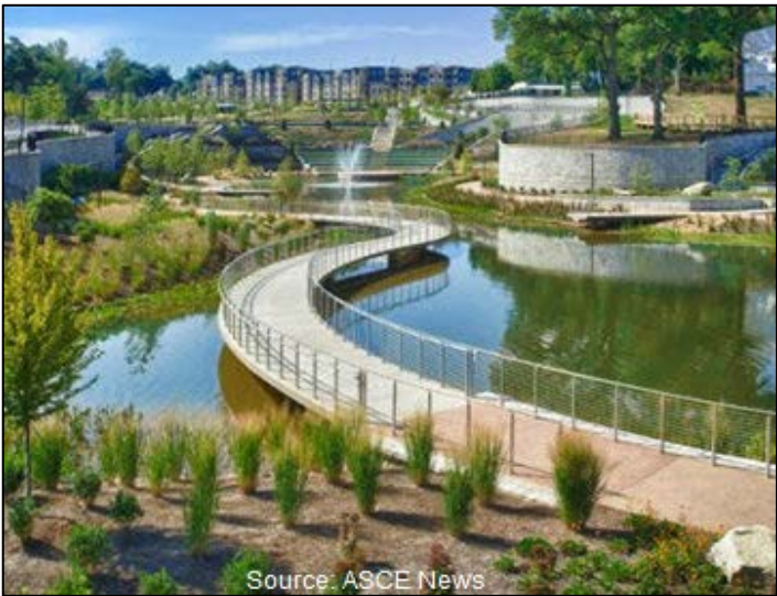
The image shows “Fourth Ward Park” in Atlanta, Georgia, a great example of this park concept. In this park, walkways traverse through stormwater ponds and native plants are used to absorb rainwater without diverting it into drains.
